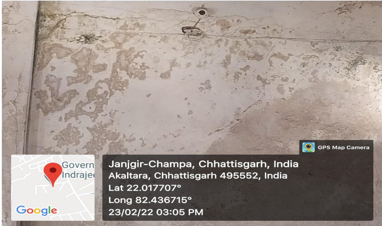
CCTV Camera in the Class
